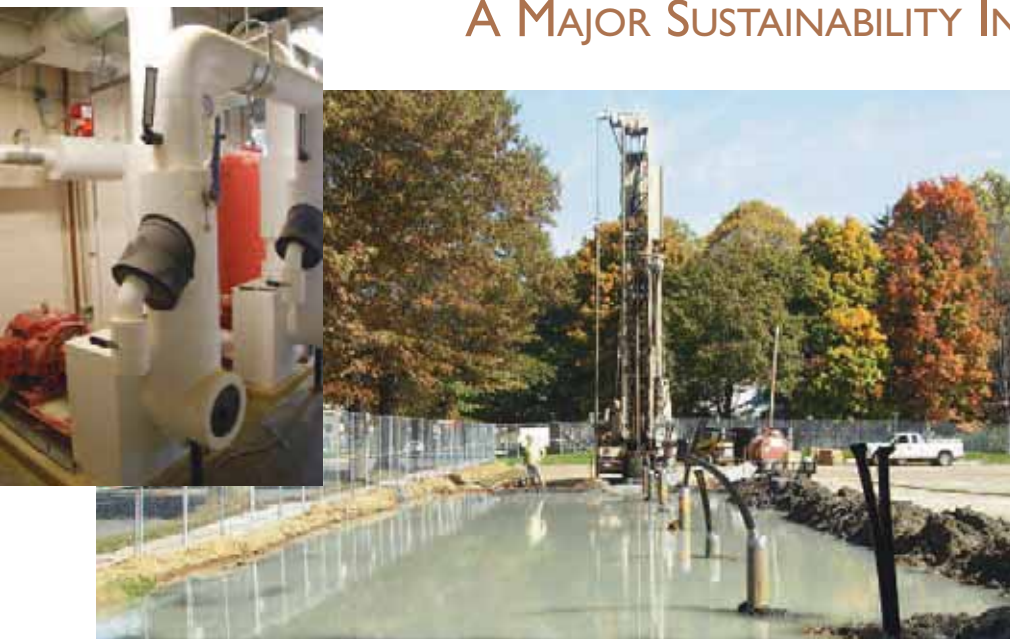
Earlier installation of wells under tennis courts.
