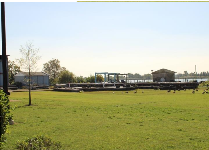
Site Photo 15: The rear yard of the Tinicum Municipal Building, with the Delaware River in the distance.
