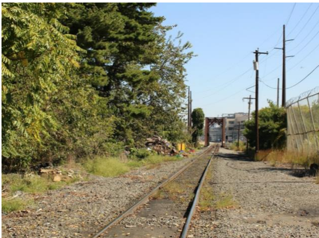
Site Photo 20: Train tracks leading into the distance.
