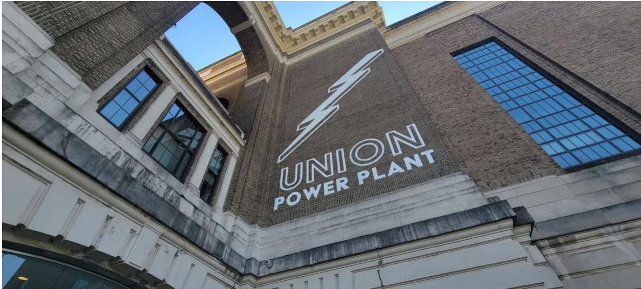
Site Photo 1: Looking up at Union Power Plant from the Main Entrance
